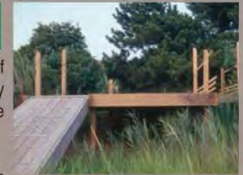
First deck on prototype pier - 1984 Lawrence, New York
