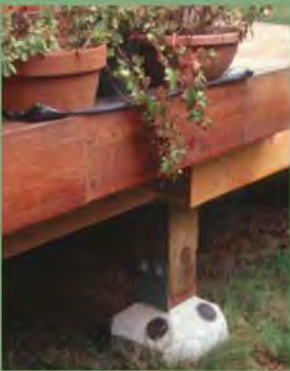
Heavy Decks, Big Timbers
