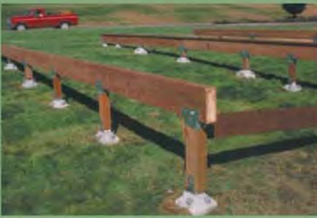
Frame Foundations for Modular Structures
